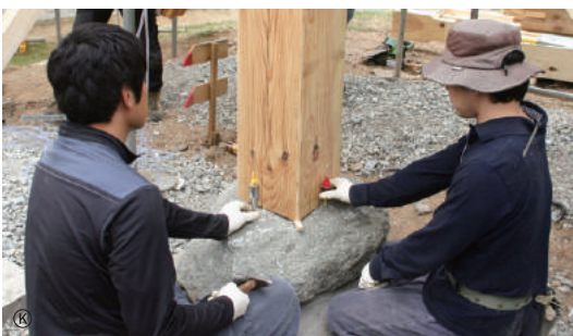
Reference column - Checking verticality and centered location
