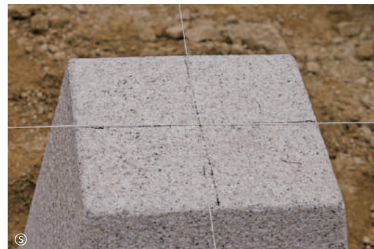
Marking the center of column base stone
