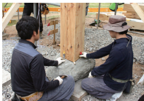
Checking verticality
