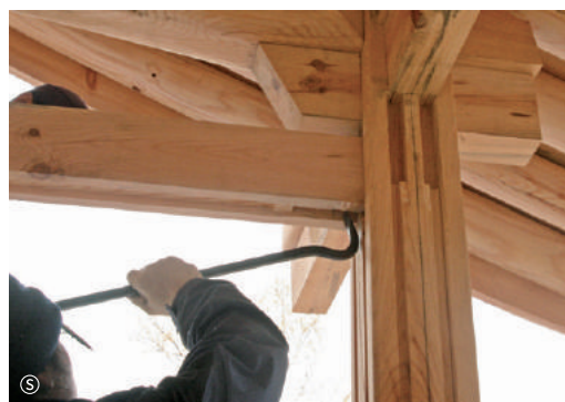
Assembling the upper lintel
