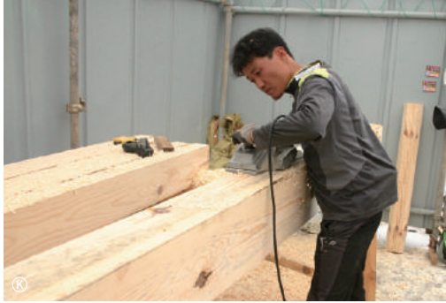
1 2 | Timberwork for column connecting beam
