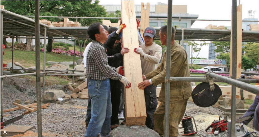
Erecting column - Marking at a certain length from the bottom end of the column
