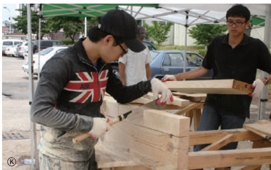
Trimming the protruding railing
