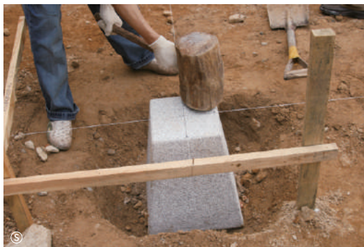
Laying the column base stone in the correct orientation
