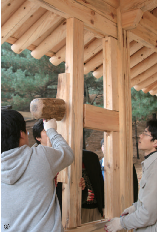
Assembling wall studs
