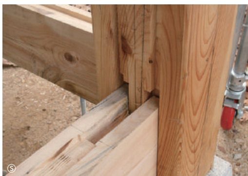
Assembling the lower lintel
