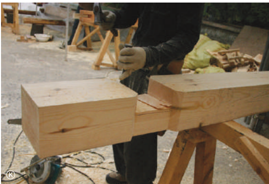
Carving mortises of the long floor joist
