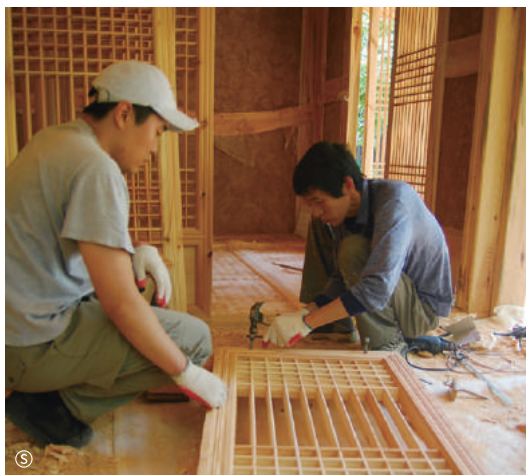
1 2 | Installing doors and windows
