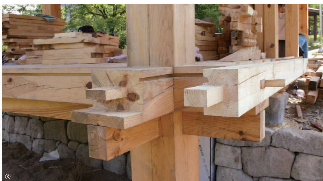
1 — 1, 2 Assembling floor joists 2
