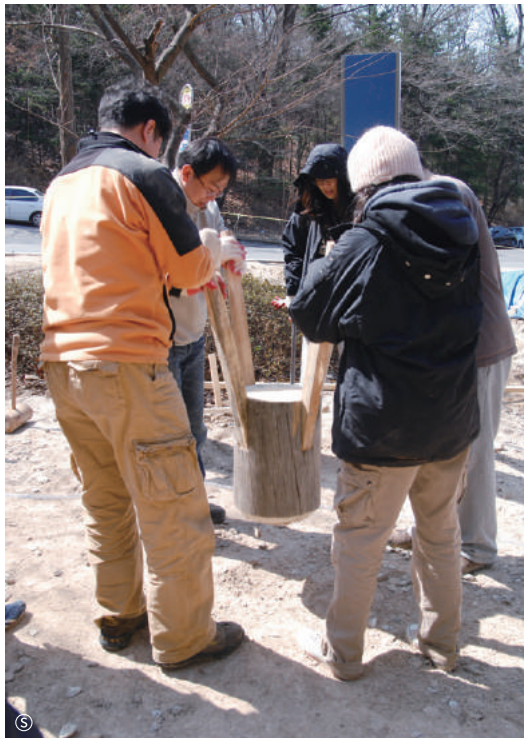
1 2 — 1 Rammering 2 Compacting 3 3 Quicklime foundation
