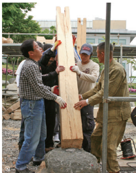
Erecting column
