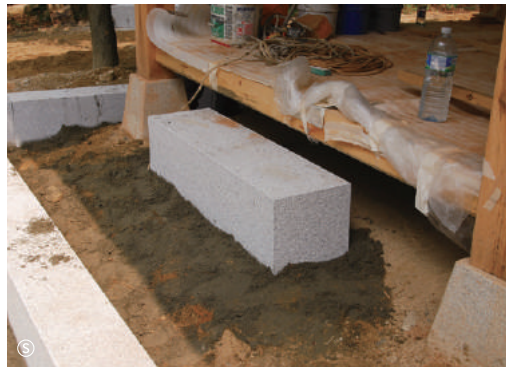
Placing the step stone
