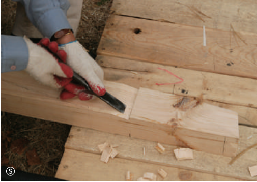
1 2 | Cutting and trimming rafters on gable board
