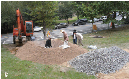
Storing aggregates and stones
