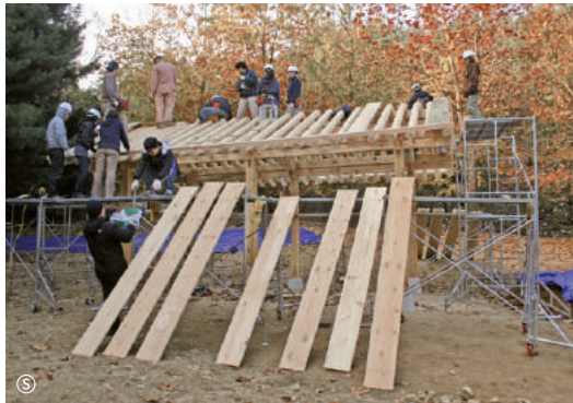
1 2 — 1, 2 Fitting rafters 3 4 — 3, 4 Placing the shingle
