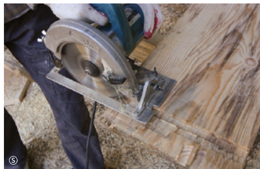
1 2 — 1 Dressing a rabbet joint for interlocking with shingles 2 Joining laths on rafters in the length direction 3 4 3 Trimming shingles 4 Dressing a rabbet joint for interlocking with laths on rafters
