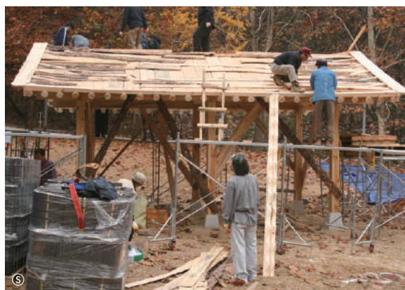
Making the roof foundation with roof filling wood
