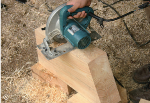
Marking and trimming truss post
